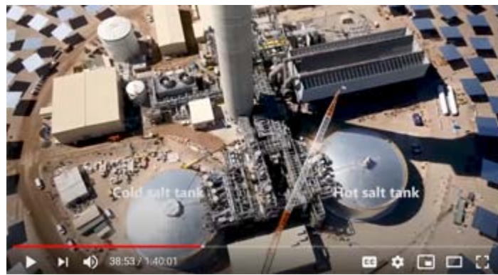
Cold salt tank / Hot salt tank Molten salt receiver]
