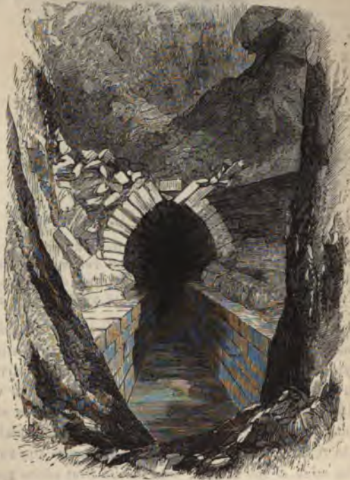
Vaulted Drain beneath South-east Palace (Nimroud)
