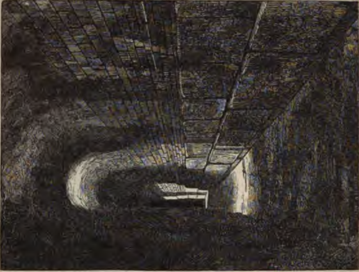
Tunnel along Eastern Basement Wall (Nimroud)
